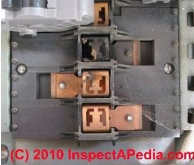
It's the exceptions that cause fires. An FPE circuit breaker will appear to "work just fine" in passing along current to the circuit it feeds, *until there is an overcurrent, short circuit, or similar condition.*
