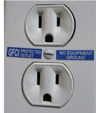
The part that makes all of this a bit more complicated is that as of January 1st, 2014, most replacement outlets in homes need to have AFCI protection. If the main electric panel in the home is too old to allow for the installation of AFCI circuit breakers, it gets really interesting. It's stuff like this that makes me really glad to be a home inspector; I get to say "have an electrician fix it". I don't have to design the exact repairs.
