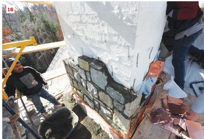
A waterproof cement-based coating (MasterSeal 581) is applied up and over the block chimney core (12). The stepped, 16-ounce copper through-flashings are fabricated and soldered on site (13). The large pieces are tacked in place with masonry anchors, and the edges sealed with polyurethane caulk (14).
