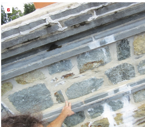
Efflorescence-stained stone veneer indicates that a lot of water had moved within the masonry chimney (6). The base flashings along the back, sides (7), and front are nailed to the face of the stone (the peeled-back caulk reveals a nail head) (8).
