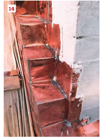
A waterproof cement-based coating (MasterSeal 581) is applied up and over the block chimney core (12). The stepped, 16-ounce copper through-flashings are fabricated and soldered on site (13). The large pieces are tacked in place with masonry anchors, and the edges sealed with polyurethane caulk (14).
