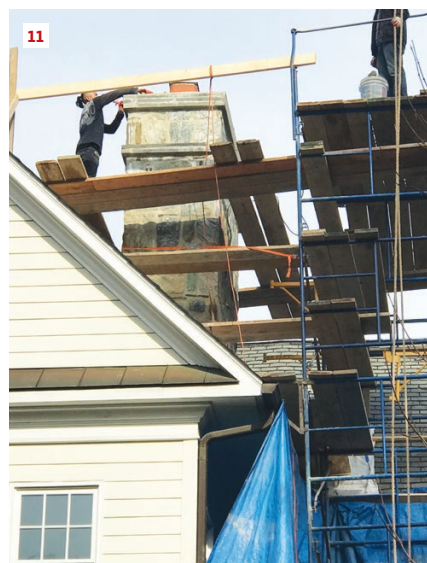
The chimney's concrete cap (9) and corbeled 1-inch-thick bluestone top are heavily caulked in an attempt to keep out moisture (10). After assembling an impressive scaffolding anchored to the building at multiple levels to provide lateral strength, the masons begin to remove the stone veneer and the cracked crown on the chimney (11).
