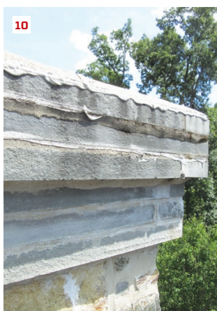
The chimney's concrete cap (9) and corbeled 1-inch-thick bluestone top are heavily caulked in an attempt to keep out moisture (10). After assembling an impressive scaffolding anchored to the building at multiple levels to provide lateral strength, the masons begin to remove the stone veneer and the cracked crown on the chimney (11).
