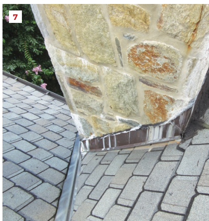
Efflorescence-stained stone veneer indicates that a lot of water had moved within the masonry chimney (6). The base flashings along the back, sides (7), and front are nailed to the face of the stone (the peeled-back caulk reveals a nail head) (8).
