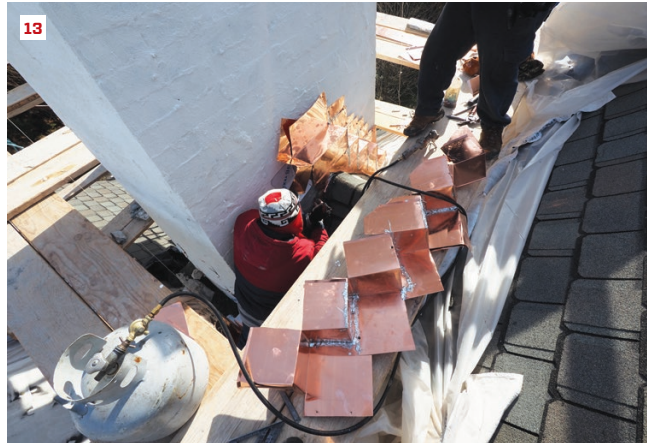
A waterproof cement-based coating (MasterSeal 581) is applied up and over the block chimney core (12). The stepped, 16-ounce copper through-flashings are fabricated and soldered on site (13). The large pieces are tacked in place with masonry anchors, and the edges sealed with polyurethane caulk (14).
