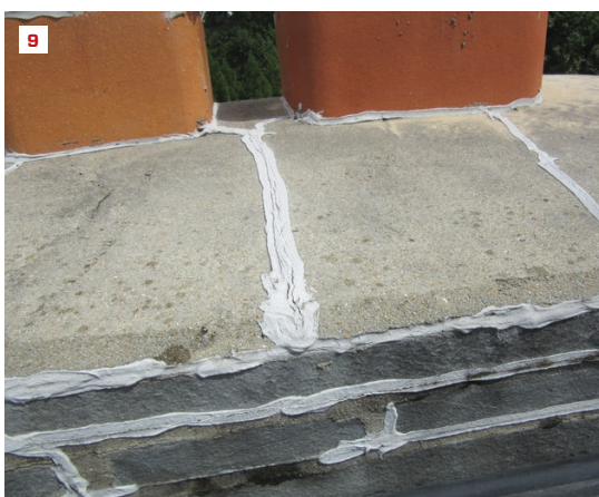
The chimney's concrete cap (9) and corbeled 1-inch-thick bluestone top are heavily caulked in an attempt to keep out moisture (10). After assembling an impressive scaffolding anchored to the building at multiple levels to provide lateral strength, the masons begin to remove the stone veneer and the cracked crown on the chimney (11).
