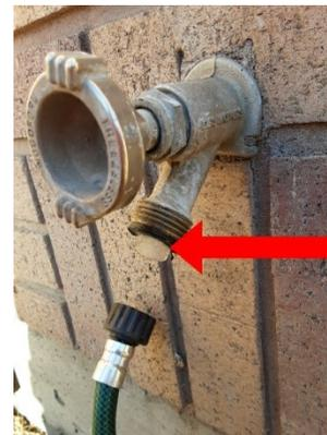
When a frost-free bib cracks during the winter, you may not even realize it until spring. When you turn that faucet on to water the lawn, pressurized water enters the cracked valve tube, and exits into the wall or floor cavity where it is installed, leading to a possibly expensive repair.
