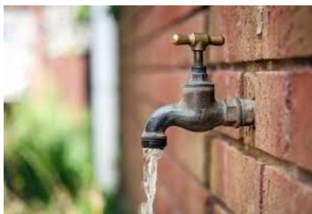
Until the late-1960’s, these units were primarily a gate valve attached to the end of a water pipe on the exterior of the home. These units were prone to freezing due to the fact the water stop point was in the cold, or un-insulated section of the home. Water would commonly freeze just inside the valve and expand the metal, usually galvanized steel, to a point that it would cause the pipe to crack.
