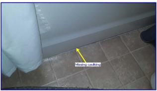
Missing or deteriorated caulking at base of tub. Recommend applying proper caulking to prevent damage to flooring.
