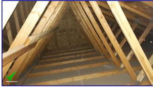
Wood truss roof structure in satisfactory condition - No structural issues observed
