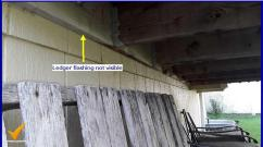
The deck ledger has no ledger flashing installed. There may be hidden damage when a deck is improperly flashed. Ledger flashing will help water to properly flow without damaging the ledger board or siding. Recommend further evaluation by a licensed contractor. Repair or replace according to deck and construction standards of best practice.
