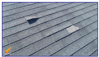
Minor wind damage on roof. Recommend having a licensed roofer repair shingles as needed.
