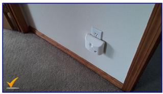
"Temporary" type Carbon Monoxide detector installed in 1st floor hallway. Although this satisfies the legality of having a functional detector, it is recommended to have mounted units installed.
