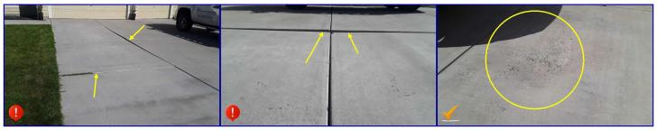
There are uneven slabs at the driveway, There are uneven slabs at the driveway, which could be a tripping hazard. Recommend using additional caution in these areas. Repair or replace as these areas. needed.
