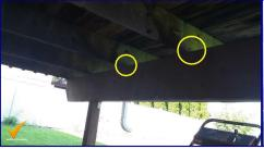
Joist to beam anchors not installed on rear deck. Recommend proper anchors be installed by a qualified professional.
