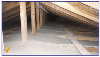
Average of 4" loose fill cellulose insulation installed over bedroom areas. Recommend additional
