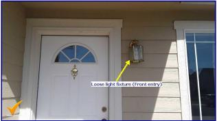
One or more exterior lighting fixtures are loose. Potential for electrical short to occur. Recommend repair or replacement by a licensed electrician.
