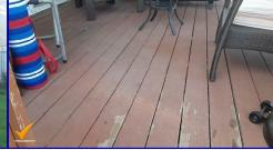
Previous deck surface coating is deteriorating and will need to be removed in order to apply new protective product. Recommend utilizing a wood penetrating stain or paint intended for exterior decking.
