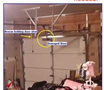
The garage door was damaged but was The garage door was damaged and not South overhead door was in functional not operable. Repair the damaged door operable. Repair the damaged door as as needed.
