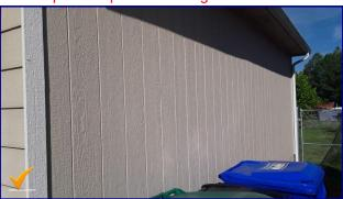
The wood siding on North exterior needs routine repair and painting maintenance. Recommend a licensed contractor to repair and paint the siding.
