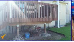
The wood in the deck needs painting or treating. Recommend painting or treating wood on the deck to help protect it from damage.
