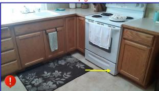
There is no Anti-Tip guard installed at the oven, which is a safety concern. Recommend a professional contractor install a tip guard.
