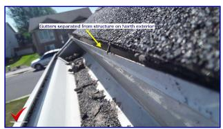
Gutters are pulling away from house on North exterior. Damage to fascia and wall structure can occur. Recommend repair by a qualified professional.
