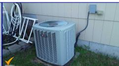
Please note; the cooling system contains R-22 refrigerant (Freon). By EPA Standards, this Freon is being phased out effective January 2020. Accordingly, when the air conditioner requires repair to the "closed refrigerant system," the R-22 refrigerant may need to be removed. R-22 may be added to the system if available, or a retrofit option may be available. We recommend saving for repairs and replacement. Consult a licensed HVAC contractor as needed.
