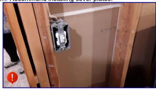
Missing cover plate on light switch to storage room. Potential safety hazard
