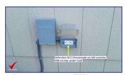
One or more exterior GFC electrical receptacles were not operational, did not trip when tested. Potential safety hazard. Recommend a licensed electrician evaluate and repair.
