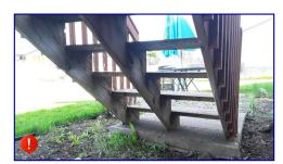
There are open risers on the exterior wood stairs, which is a potential safety concern. Recommend using additional caution in these areas. Install proper risers for added safety.
